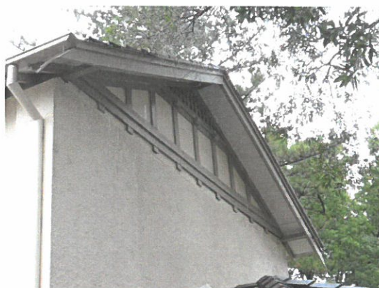
Figure 3.21 The eastern gable of the chapel wing. The shadow in the stucco below shows the location of the window that was originally located in this wall. (Source: GML 2017)
