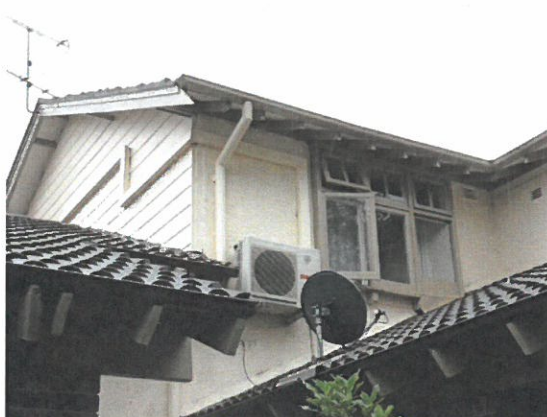
Figure 3.17 The original timber window that exists in the upper part of the east elevation of the main part of the building. The boarded gable of the south elevation can be seen on the left. (Source: GML 2017)
