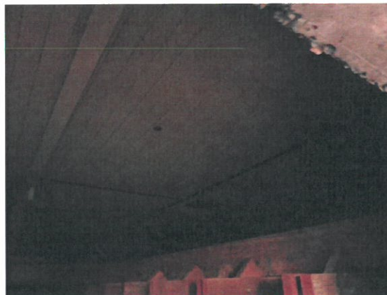
Figure 3.46 The original boarded ceiling remains above the newer cedar ceiling in the chapel. The dark lines possibly indicate the former location of walls. (Source: GML 2017)
