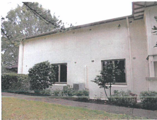
Figure 3.18 The north (front) elevation of the chapel wing. 'Shadows' of former window openings can be seen in the stucco finish. (Source: GML 2017)
